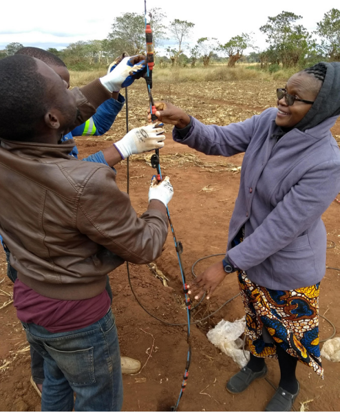
Figure 3 Sensor installation in boreholes at the Chitedze site near Lilongwe. Arrays of sensors are being lowered into hand-augered boreholes.
