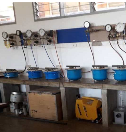
Figure 5 New CEPHaS equipment installed at the University of Zambia.
