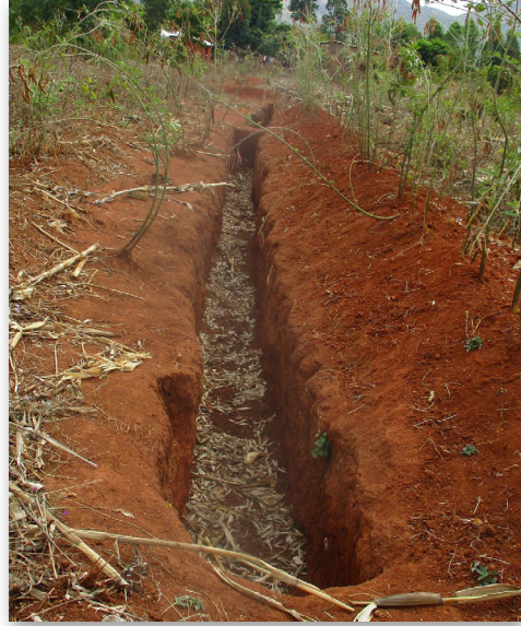
A modified water absorption trench in an agricultural field is fortified with pigeon peas planted on the overflow embankment (Source: Bascom et al. 2021).
